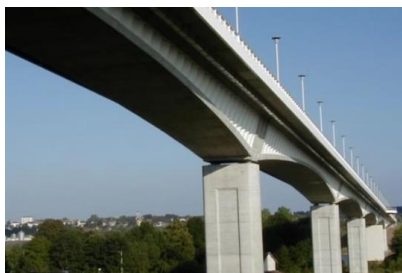
(a) Dole bridge girders with CWs, France
